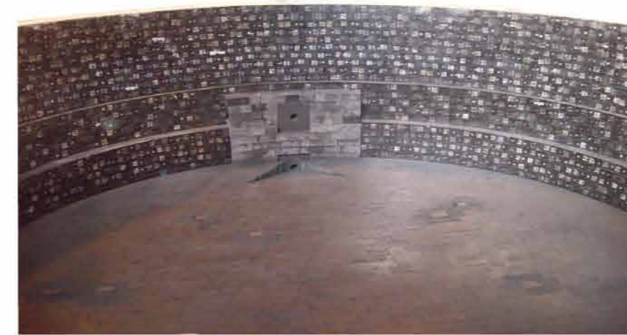
● 電爐耐火材料施工 Construction of EAF Refractories.
