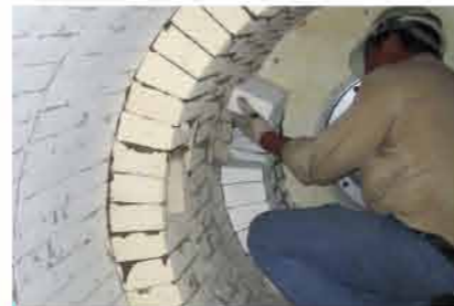
● 圓筒型窯爐施工 Construction of Cylinder furnace.
