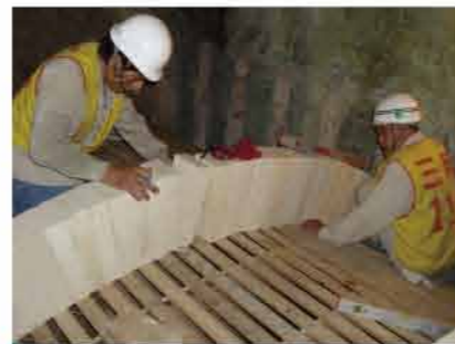
● 窯爐拱磚施工 Construction of furnace' s arch bricks.
