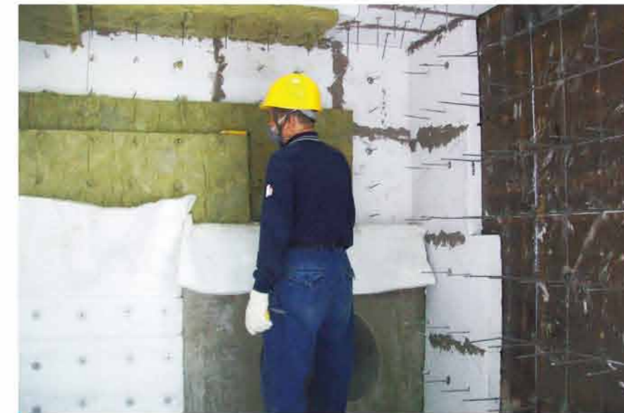
● 保溫材料(棉毯)施工 Construction of Insulating Material (blanket).
