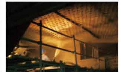
● 爐頂噴漿施工 The gunning of EAF Roof.
