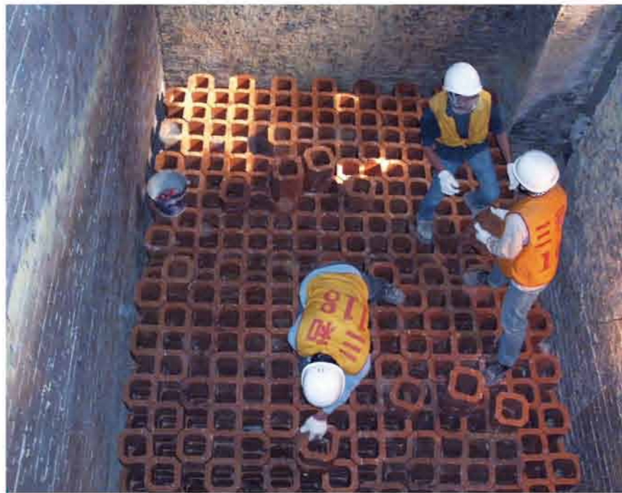
● 玻璃窯爐蓄熱室磚施工 Construction of the regenerator of glass furnace.
