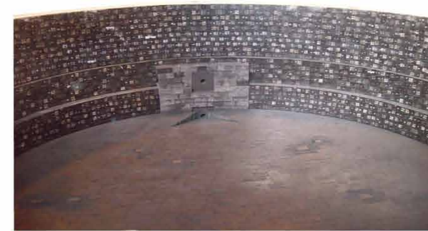
● 電爐耐火材料施工 Construction of EAF Refractories.
