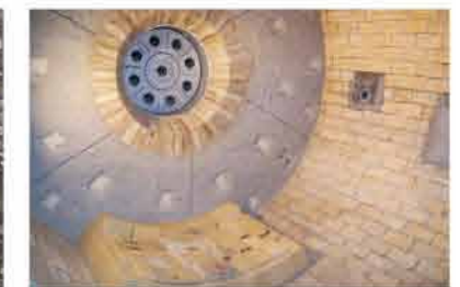
● 砌磚與搗固施工完成圖 Brick Installing and Ramming Constructure.
