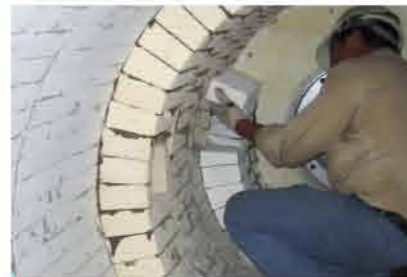
● 圓筒型窯爐施工 Construction of Cylinder furnace.
