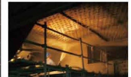
● 爐頂噴漿施工 The gunning of EAF Roof.
