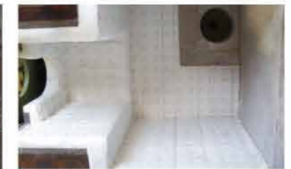
● 保溫材料施工 Construction of Insulating Material.
